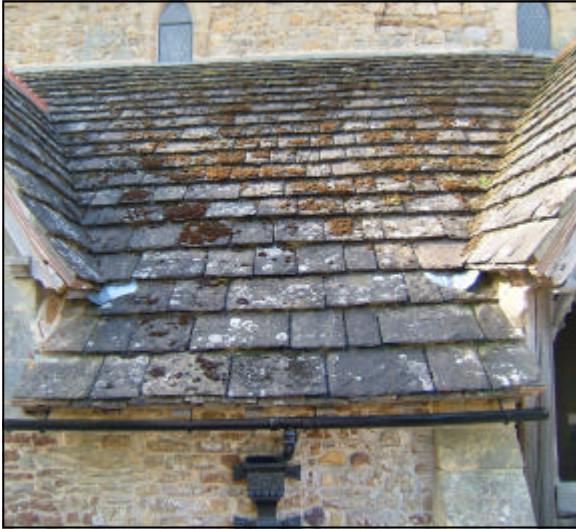
Figure 10. The first choice for the roof covering should always be Horsham stone. This will usually be a condition of any grant.
