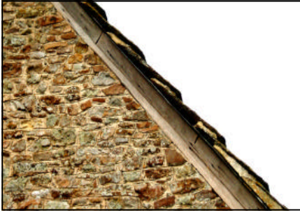
Figure 17 Verges are commonly bedded onto a slate undercloak but the mortar often falls out. If the bedding cannot be struck off as slating progresses it should be left well set back or raked out so that there is a good key for pointing up.
