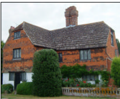
Figure 13 Hips are not very common on Horsham stone roofs but are often seen on gables and dormers.
