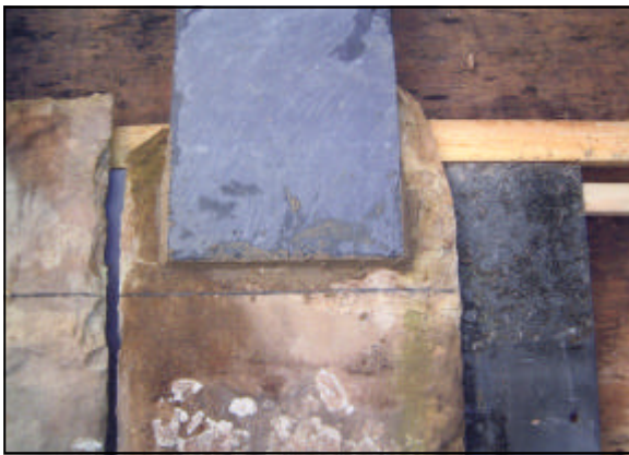
Figure 6 Shadow in position and mortar trimmed off at the edges.
