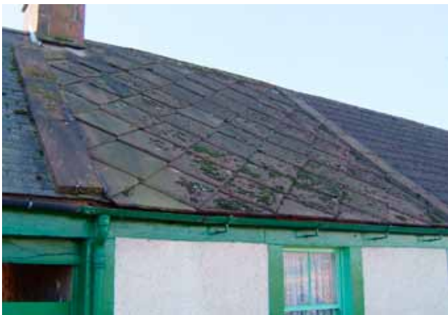
Diamond pattern. New Red Sandstone slates in Dumfriesshire
