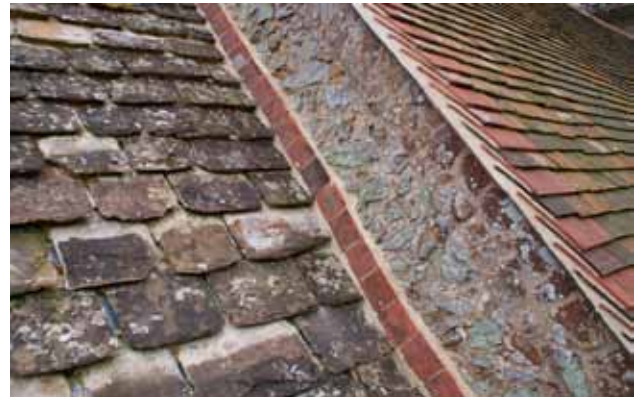
Listing Clay tile listing on a Horsham stone roof
