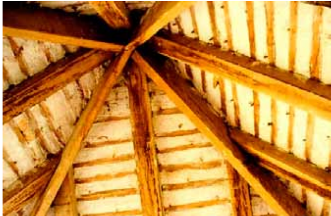
Torching Full torching in a Cotswold roof.
