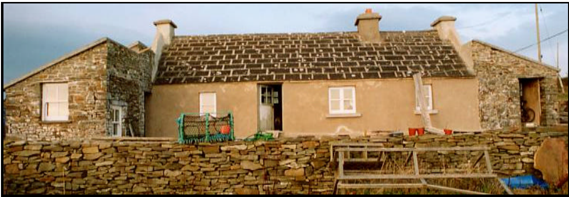
Figure 12: View of stone roofed house in NW Clare undergoing conservation work
