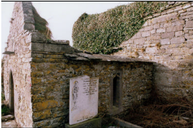
Figure 4: Kilmacreehy church, Liscannor, view of 16 th century porch. Note stone slates capping sidewall.
