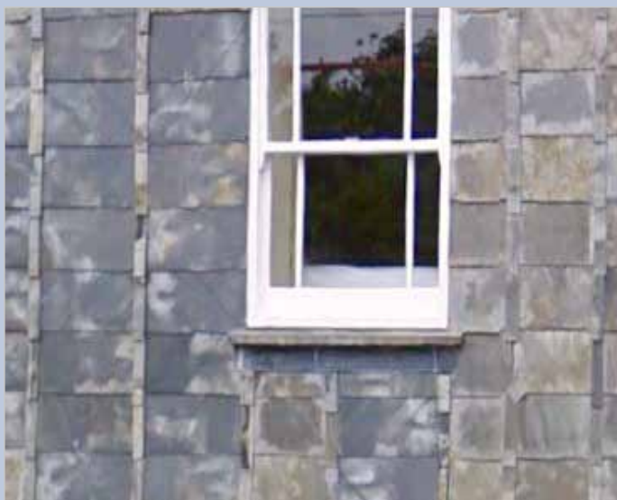
PATENT SLATING IN CORNWALL
