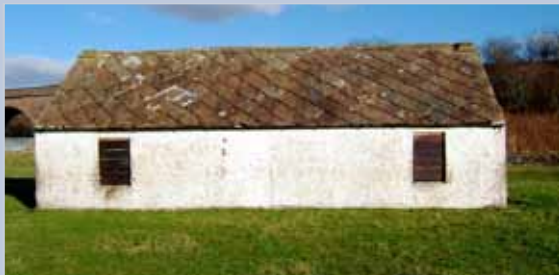
DIAMOND PATTERN SLATE AND STONE IN DUMFRIESHIRE
