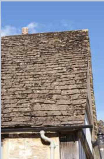
TRIPLE LAP CORNISH SCANTLE SLATING TINTAGEL
