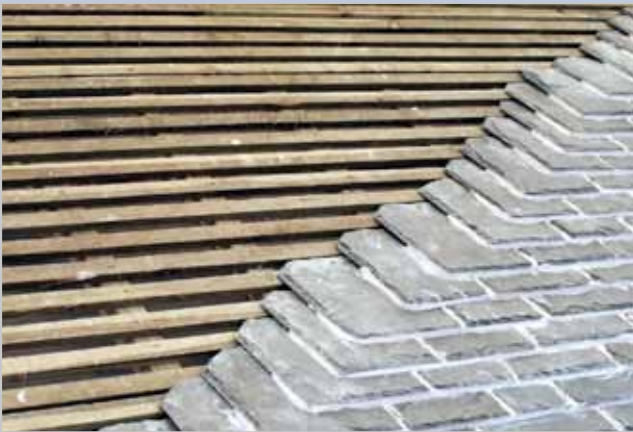
CORNISH WET LAID TRIPLE LAP DEVON SCANTLES
