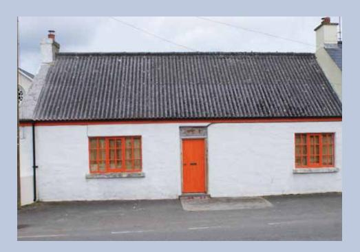
**Profiled sheets** are in effect very large pan tiles but are also profiled in the 'pan' to be self supporting. They are mitred at the corners in the same way as tiles.
