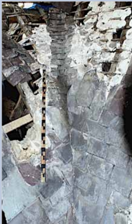
The mitred slates have been removed in the upper section to reveal the valley slates.
