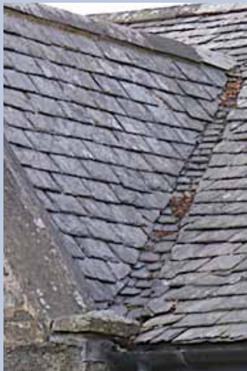
The mitred slates have been removed in the upper section to reveal the valley slates.
